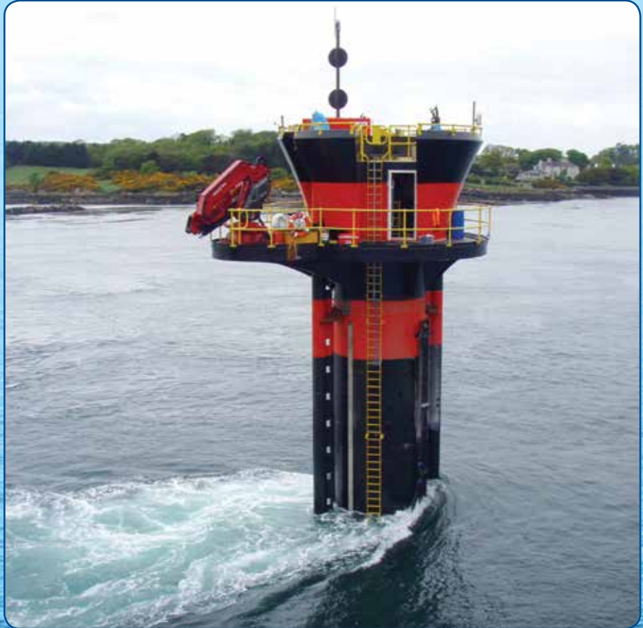
Image courtesy of Marine Current Turbines Ltd.
